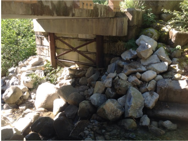
Right Bank Abutment when facing downstream
