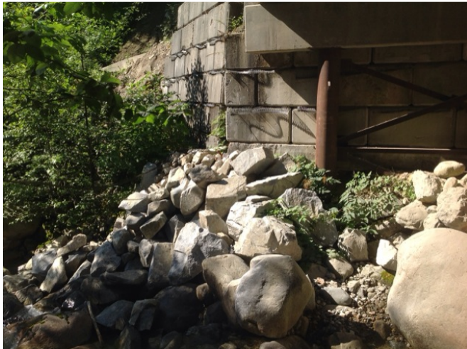
right downstream wing wall
