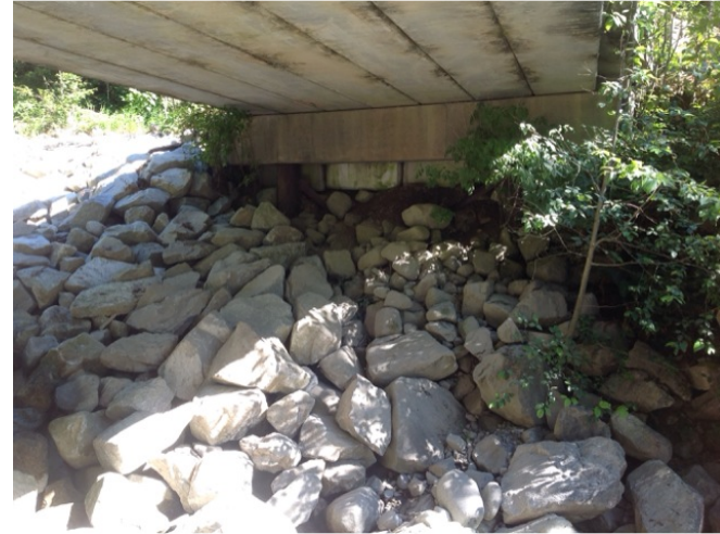
Left Bank Abutment when facing downstream
